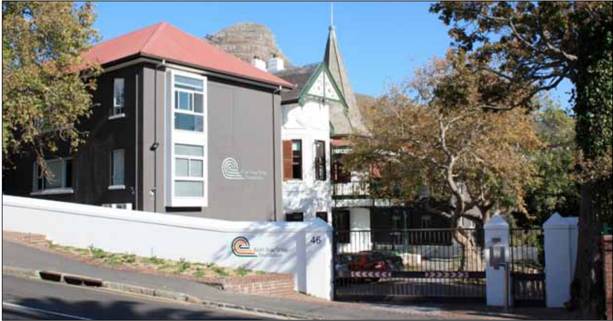
The Foundation's new offices are located at 46 Hof Street, Oranjezicht, Cape Town, 8001. Contact numbers: (T) 021 481 5400 (F) 021 086 554 0000.
